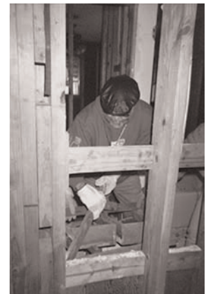
Charles Marks tears out a mold-damaged bathroom
